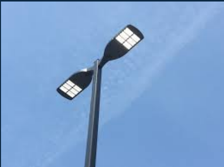
Shoe box type fixture in parking area
