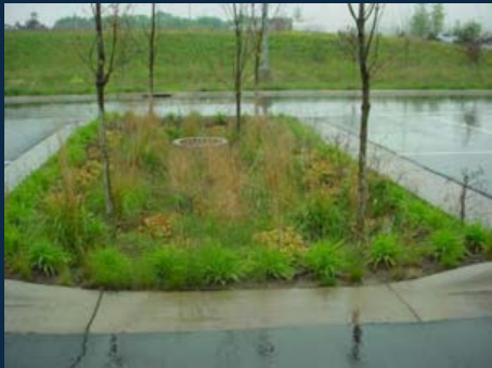
Parking island with ribbon curb for use as storm water BMP / rain garden
